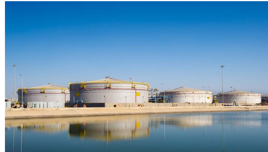
Rajasthan: Mangala Processing Terminal
