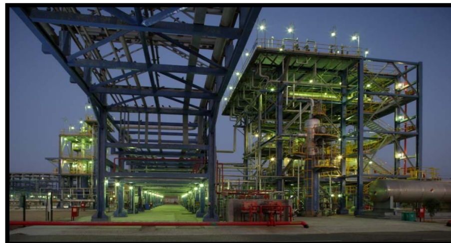
Rajasthan: Raageshwari Gas Terminal
